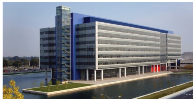
General Motors Technical Center
